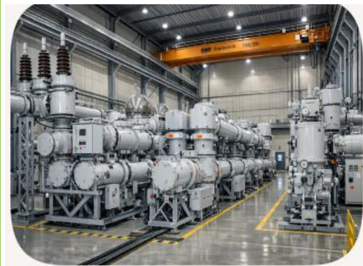
Figure 4: 400KV GIS Indoor configuration
