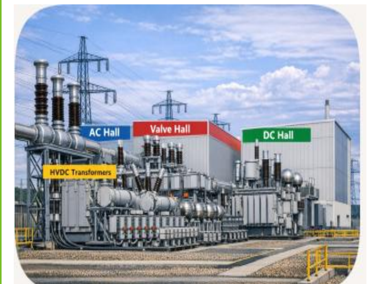
Figure 6: Onshore Converter Station Overview
