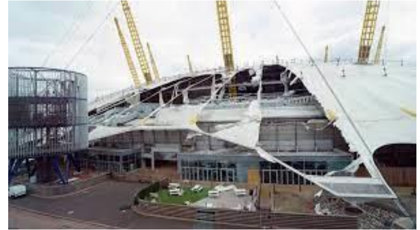
Storm Eunice wind damage
